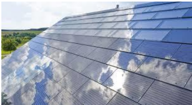
Placing of a solar power plant on the territory of v. Stryzhavka, Vinnytsia region
