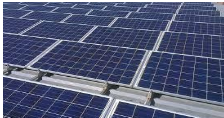
Building of a solar power plant on the territory of v. Zhabelivka, Vinnytsia district
